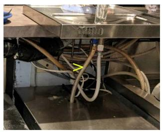
The yellow arrow points to the spill tray drain line. Using braided vinyl for drain lines is not recommended. Besides costing slightly more than un-braided, you can't see through it. Seeing build-up inside that line creates a sense of urgency to get it changed. If only draught service techs understood this, they'd sell more drain line and you'd have fewer fruit flies.
